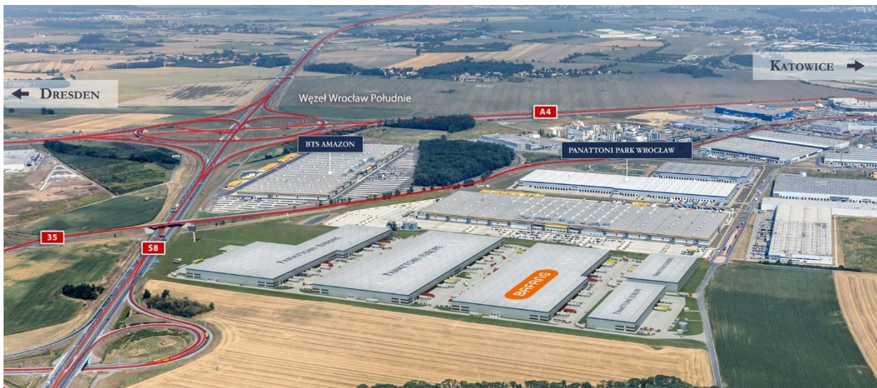
Aerial view of 'Panattoni Park Wrocław' industrial zone
